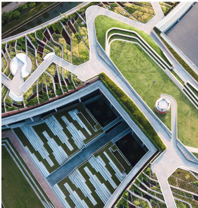
TWA Thailand Government Complex © Kotchakorn Voraakhom
